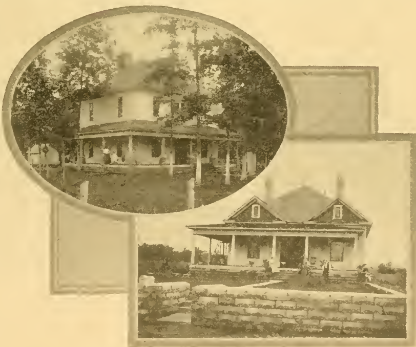
FARM HOUSES IN JEFFERSON COUNTY
